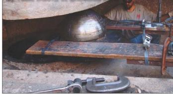
The moment of truth as the custom-made pintle ball is moved into place under the dam gate. There were no existing replacement parts available for this work at Chouteau Lock and Dam 17 in Chouteau, Oklahoma, so crews were forced to wait until the actual placement of the part to know if it would fit, which it did.
